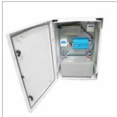
UPS (Uninterruptible power supply) Run the sign on battery during the day and charge it on the trafficlight during the night.
